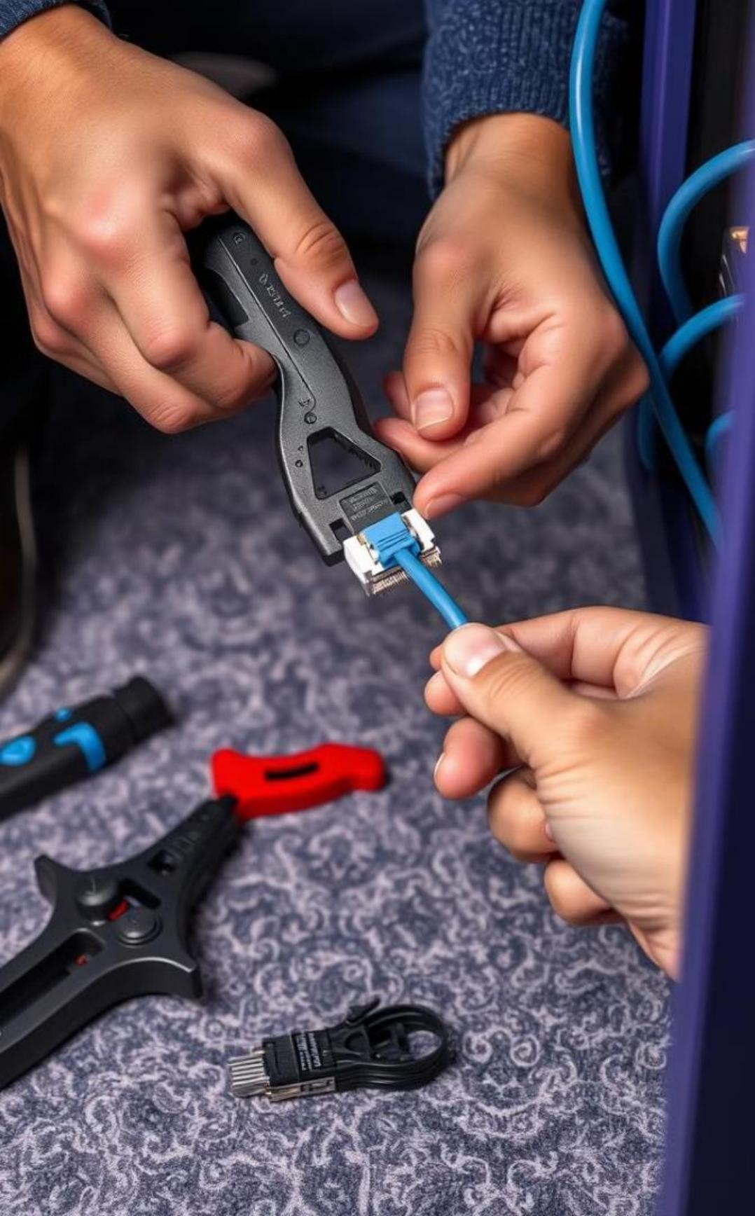
A close-up photograph showing a person's hands using a black crimping tool to attach a blue Ethernet cable to an RJ-45 connector. The person is wearing a blue sweater. In the background, there are other blue Ethernet cables. In the foreground, there is a blue patterned surface with various tools including a red-handled screwdriver, a black crimping tool, and a black Ethernet cable with a RJ-45 connector.
